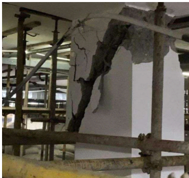
柱受剪裂缝
